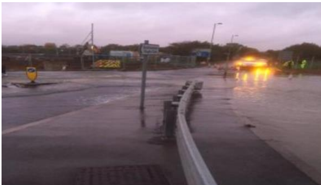
Figure 3: Significant flooding on Brownhill Way, an arterial route from the M27 to Southampton city centre.
