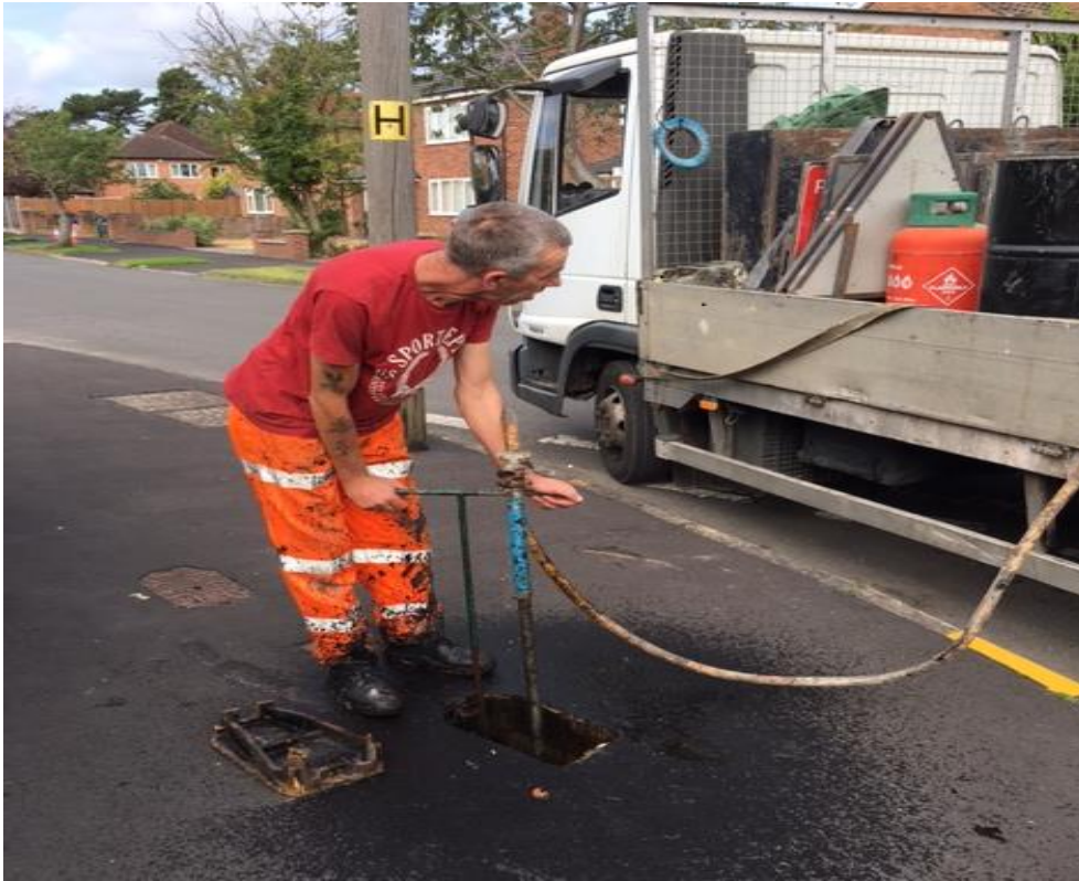
Figure 5: Unlicensed, ill-fitting and unhygienic use of hydrants is not only theft of water but puts consumers at risk from discolouration and contamination. The company was successfully prosecuted by Severn Trent Water
