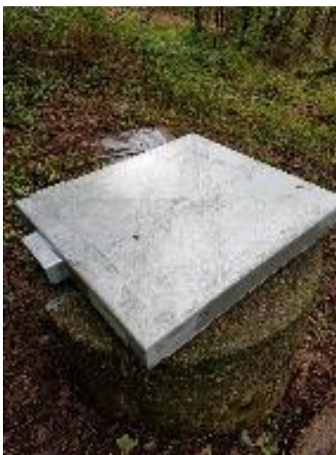
Figure 5: Replacement Technocover on the spring source at Hook works
