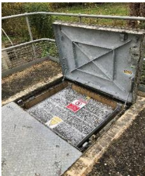
Figure 4: Perspex cover to protect operators at Rodbourne works
