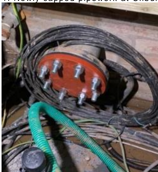
Figure 1: Newly capped pipework at Cliburn works
